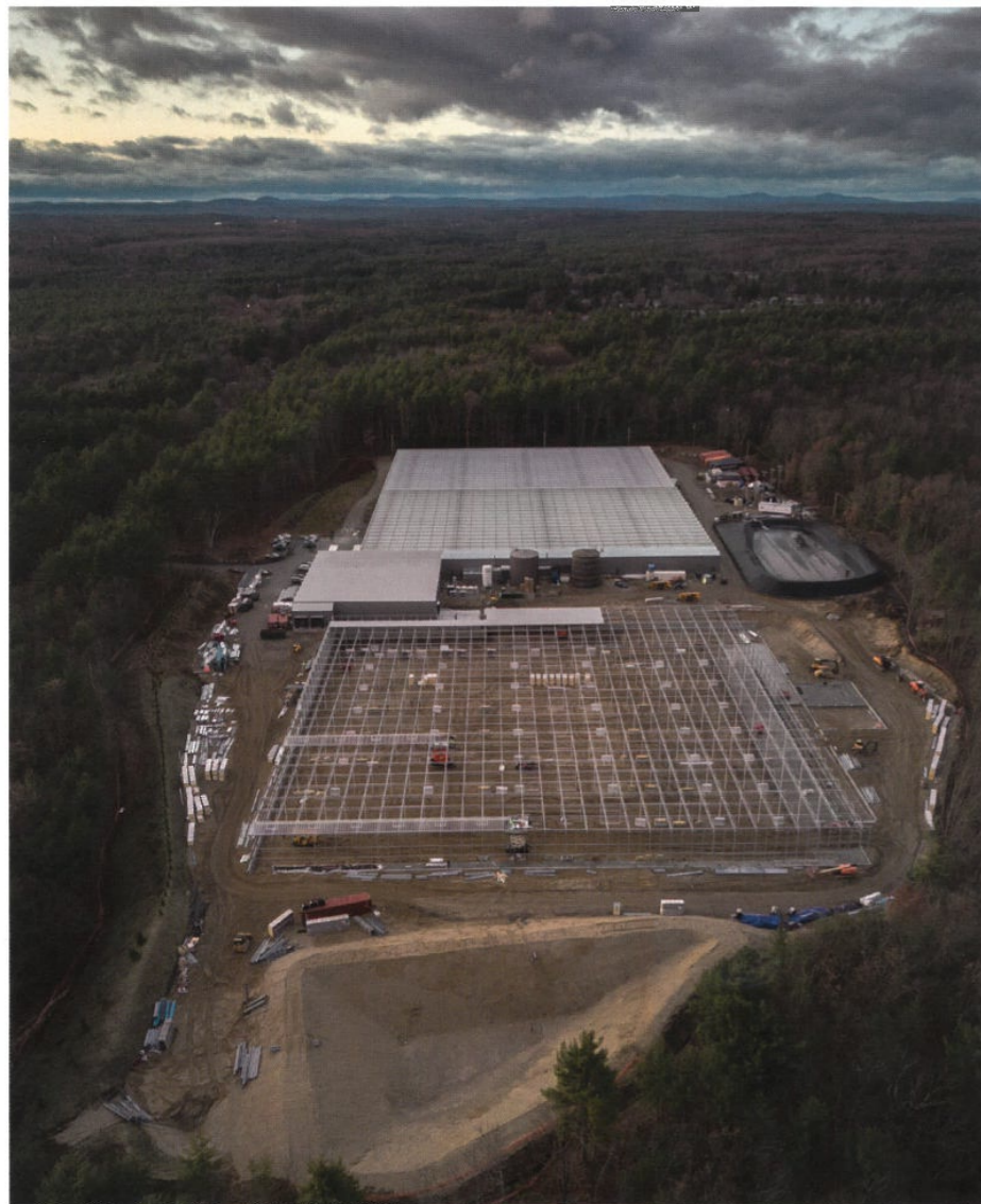
Phase 2 (middle) was added after just one year, doubling the size of the greenhouse. Phase 3 (bottom) was completed in April 2020.
